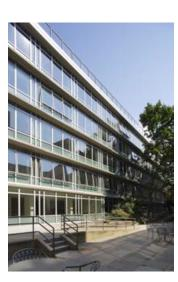
Part of the Advantage by Wausau standard product offering, the 3250iH Heritage Series 3.25-inch-deep aluminum frame, casement windows were chosen to replace the existing windows, many of which were more than 40 years old. In addition to providing residents with plenty of daylight and stunning views of downtown Philadelphia, the windows offer residents natural ventilation, an important feature given KCECH's lack of air conditioning in residential rooms.
