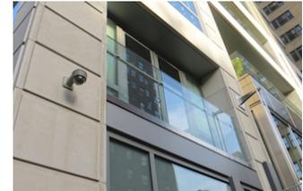
Contributing to the project's durability and cohesive aesthetics, Linetec finished the windows' and doors' 4.5-inch-deep aluminum frames in a three-coat 70 percent PVDF resin-based coating. A custom Pewter color was used. The screens were painted to match.
