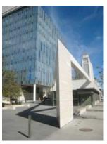
Contributing to the building's intended longevity, the window and curtainwall systems also were tested to meet stringent performance criteria. Seismic performance was of particular concern as the previous police administration building, constructed 1955, and was not expected to withstand another moderate earthquake.
