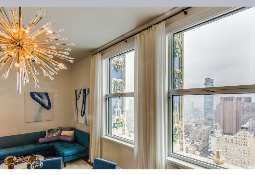
The windows on the Woolworth Tower Residences' top 30 floors featured, double-hung units manufactured using non-thermal framing and 1-inch insulating glass without the low-e coatings available today. Floor-by-floor, the multi-phased window retrofit project was successfully completed with Wausau Window and Wall Systems' 4250i INvent Series Simulated Double-Hung Projected high-performance windows.
