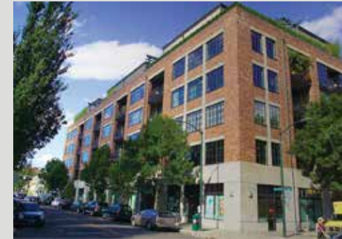
McKenzie Lofts . Obsidian Architecture
