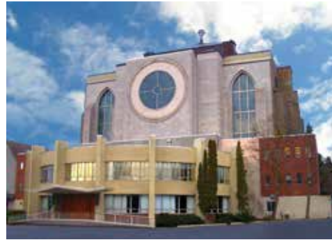
Saint Mark's Episcopal Cathedral . Olson Kundig
