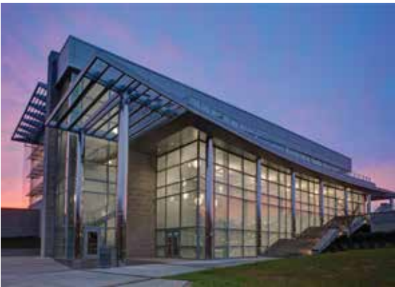
Engineering and Math Building at Cecil College . Marshall Craft Associates
