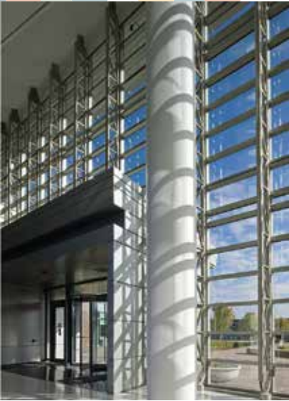
Sheppard Hall at Joint Base Andrews . AECOM
