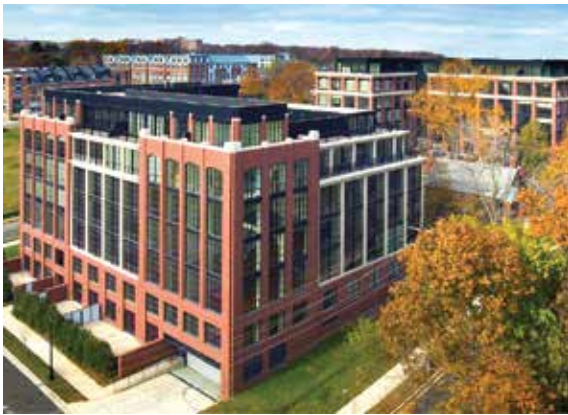
Wooster and Mercer Lofts . Cunningham Quill Architects
