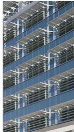
Exterior sun shades and re-cladding
