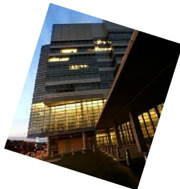
In strictest architectural parlance, a **“curtainwall”** is any non-load-bearing exterior wall that hangs, like a curtain, from the face of floor slabs, regardless of construction or cladding material. However, in common usage, the term curtainwall usually refers to aluminum-framed systems carrying glass, panels, louvers, or occasionally, granite or marble. Curtainwall supports only its own dead load.
