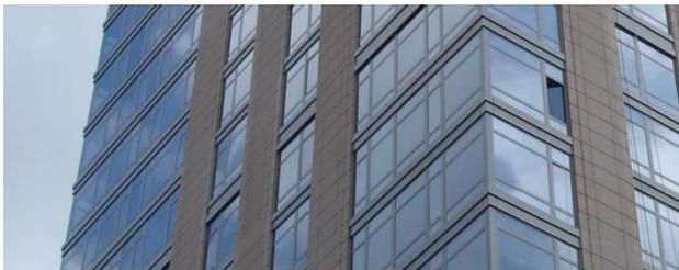
“**Window wall**” spans from the top of one floor slab to the underside of the slab above.
