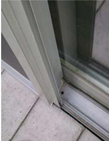
Permeable decking can allow the use of weather-able sills and a curb under an accessible threshold
