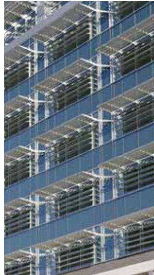
Exterior sun shades and re-cladding
